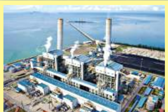
Sultan Azlan Shah power station in Manjung, Perak (Energy source: Coal)
