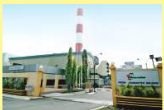
Gelugor power station in Pulau Pinang (Energy source: Diesel)
