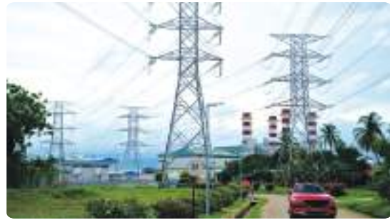
132 kV alternating current transmission cables at the Tanjung Kling Power Station, Malacca
