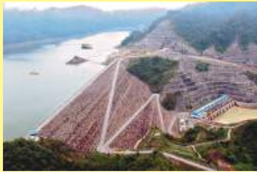
Bakun hydroelectric power station in Sarawak (Energy source: Hydro energy)
