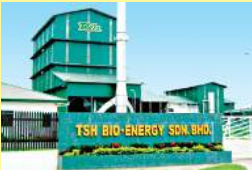
TSH Bio-Energy Sdn. Bhd. Biomass power station in Sabah (Energy source: Biomass)
