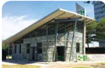
Photograph 10.11 Cyberjaya Community Recycling and Collection Centre
