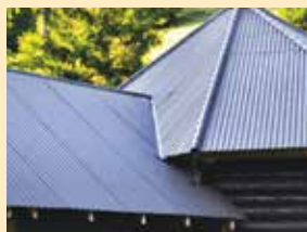
Galvanised iron roof
