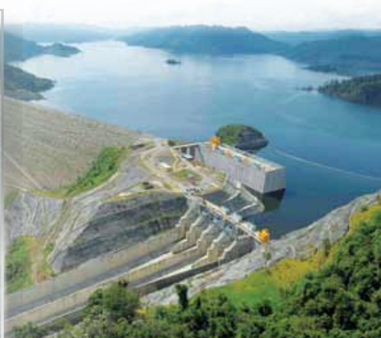
Photograph 6.3 Hydro dam in Bakun, Sarawak
