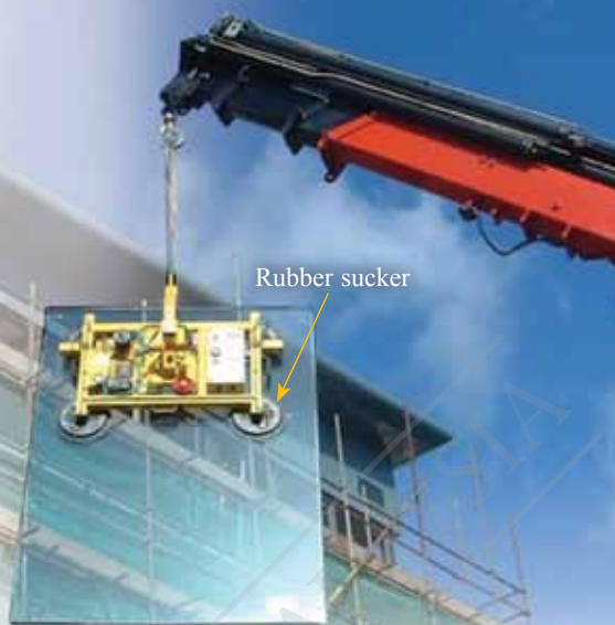
Photograph 2.2 Glass sheet lifted using large rubber suckers
