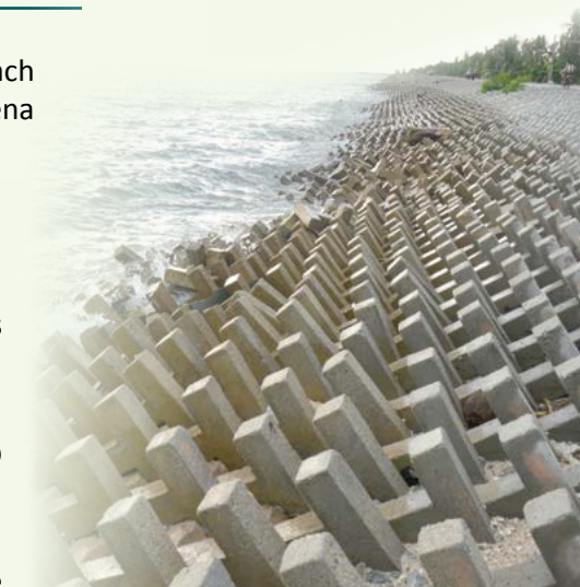
Photography 6.5 Seawalls along the coast in Tanjung Piandang, Perak
