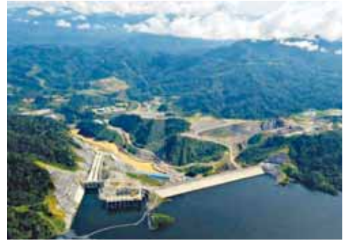
Photograph 3.5 Bakun hydroelectric power station
