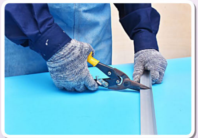
4 Memotong bingkai aluminium.
