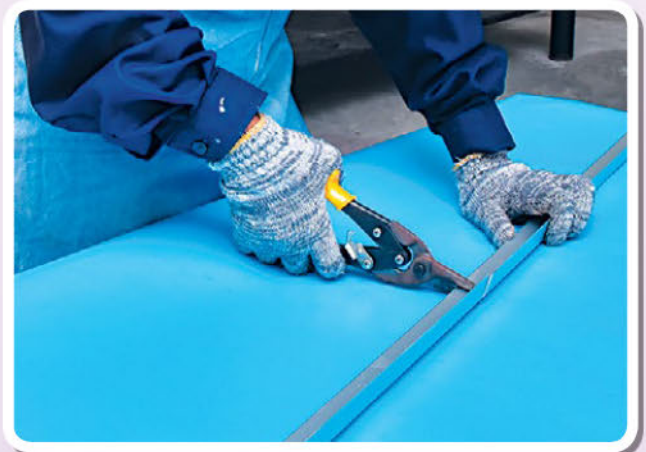
4 Memotong bingkai aluminium.
