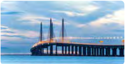
Sultan Abdul Halim Muadzam Shah Bridge 24 km
